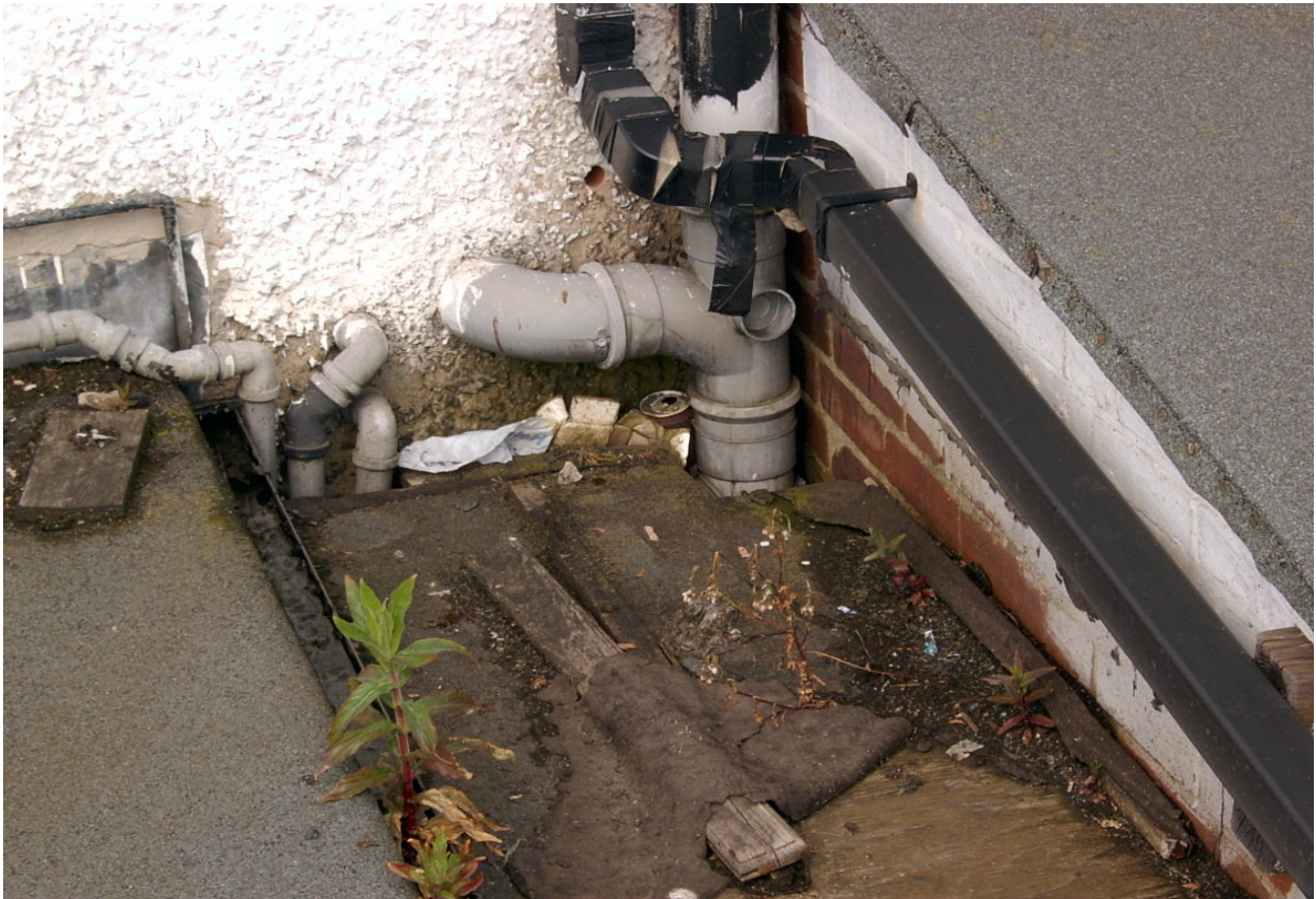
Photos 2 & 3 – Here we would describe the condition of the structural elements.
